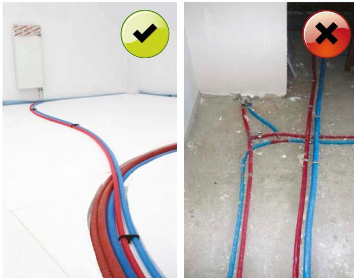
**To eliminate the excessive load on fittings by bending force, it is not recommended to bend pipes at a distance less than 10 external diameters from the fitting.**
