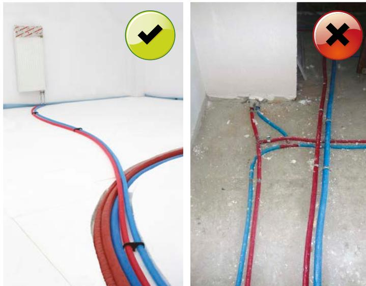
To eliminate the phenomenon of excessive fittings mechanical load with bending force, it is forbidden to bend pipes at a distance of less than 10 external diameter from the fitting itself.
