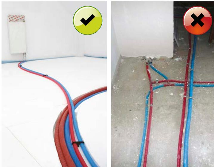
To eliminate the phenomenon of excessive fitting mechanical load with bending force, it is forbidden to bend pipes at a distance of less than 10 external diameter from the fitting itself.
